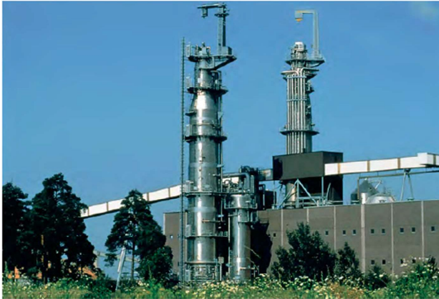
Figure 1: Alloy 2205 Continuous Sulfate Pulp Digester and Impregnation Tower
