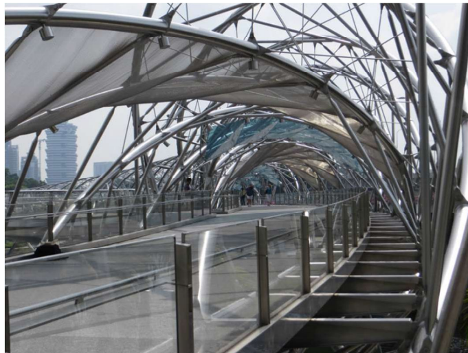
Figure 5: Marina Bay Pedestrian Bridge, Singapore
