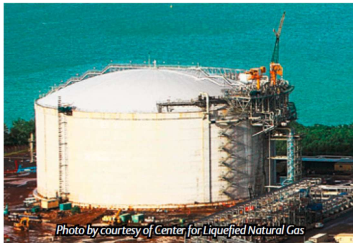
Figure 4: Cryogenic Tank Storing LNG at -260°F
