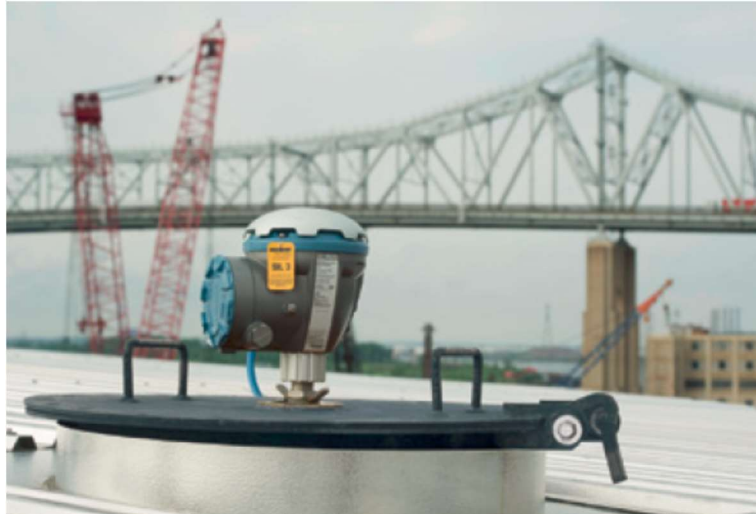
Figure 12: Modern radar level gauge on a fixed roof tank
