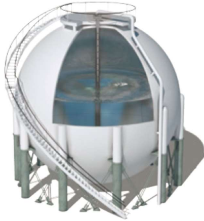
Figure 3: Pressurized tanks normally require automatic tank gauging in a still-pipe
