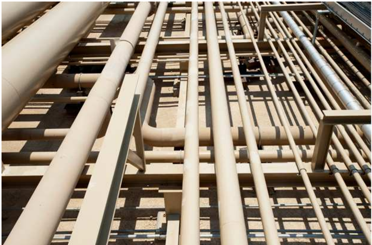
Figure 4. Pipes made of SA-106
